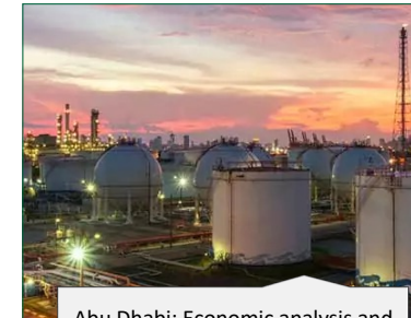
Abu Dhabi: Economic analysis and measurements for EPC Trakker refinery waste treatment plant
