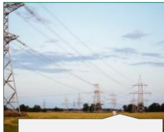
Ukraine: Power Transmission Utility Sustainable Development
