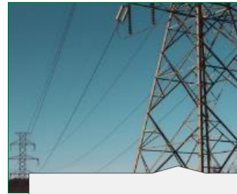
Tanzania Rural Electrification Expansion Program (OE)
