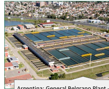
Argentina: General Belgrano Plant - New raw water lifting station 1st Stage
