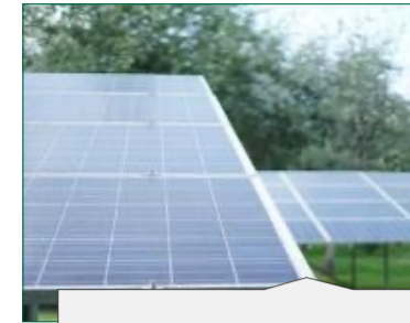
The Gambia: Owner's Engineer and Capacity Building for 8 MWh BESS.
