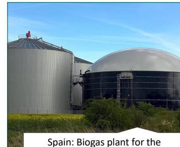
Spain: Biogas plant for the production of biomethane and compost, located in the municipality of Noez (Toledo)
